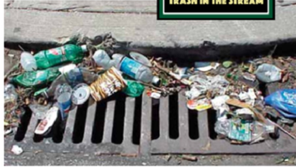
Trash accumulates and clogs a storm drain. Some of this trash will end up in our local waterways.
